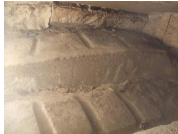
On the upper face of the beams being much higher than wide, lashing grooves have been dug to ensure stability.
