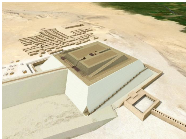
Aspect of the pyramid in the 2007 version during the construction of the 3rd ceiling. The construction site of the volume is suspended in periphery at the level +43m.
