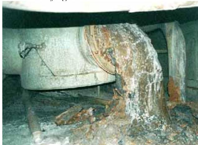
Figure 6 – Lava in steam discharge valve of SDC
